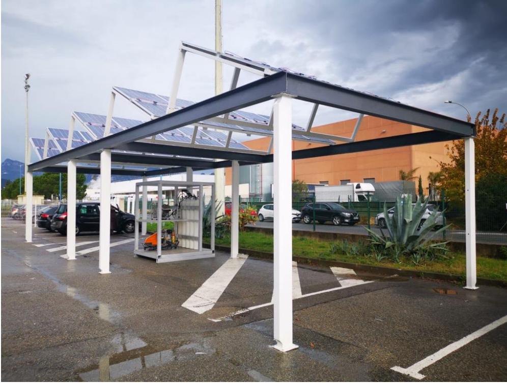
MDI AirLab solar panels and storage bottles.
